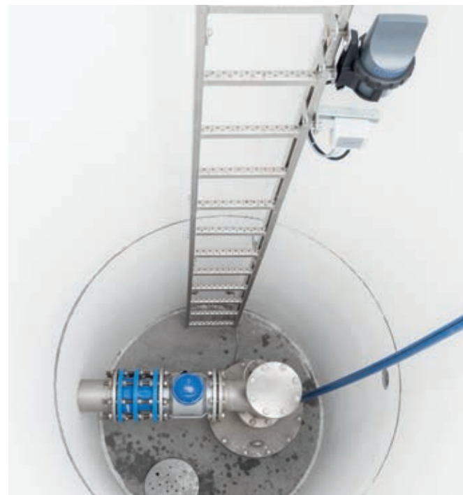
Battery-powered IP68 metering point with GSM/GPRS communication
