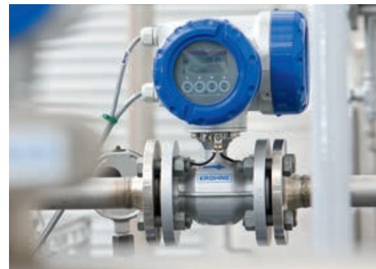
Virtual reference for EMFs: grounding rings made redundant
