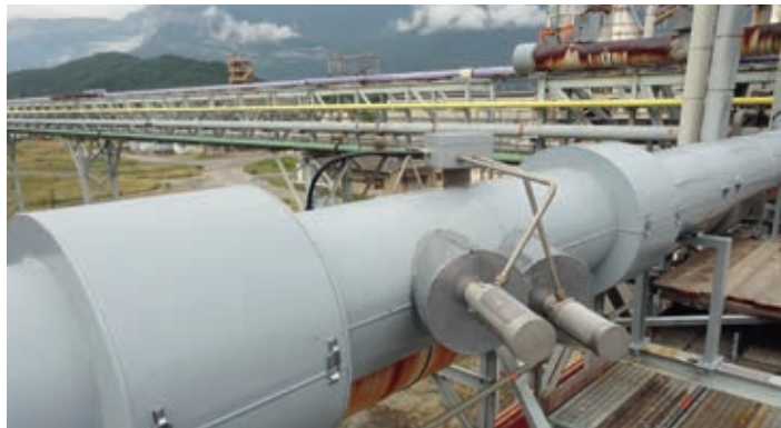
Ultrasonic flow measurement of superheated steam
