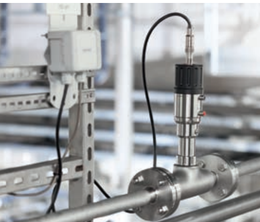
Manual retractable assembly for a pH sensor in a chemical plant
