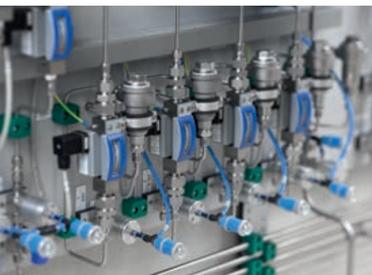
Inertisation with purge meters
