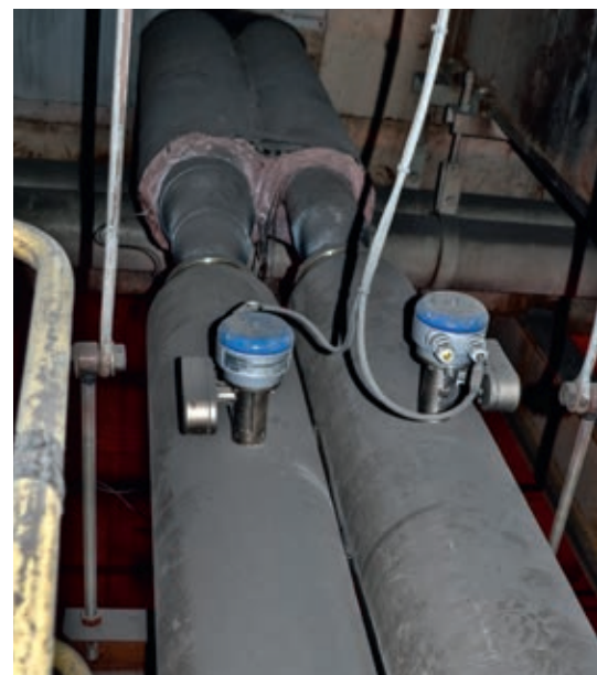
Mass flow measurement of heavy fuel oil
