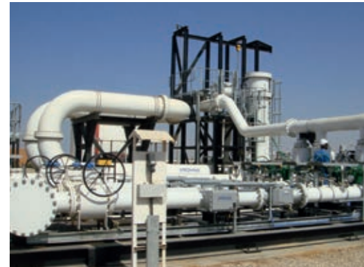
Skid mounted metering system with integrated ball prover
