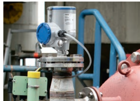
Butanol level measurement on bypass chamber
