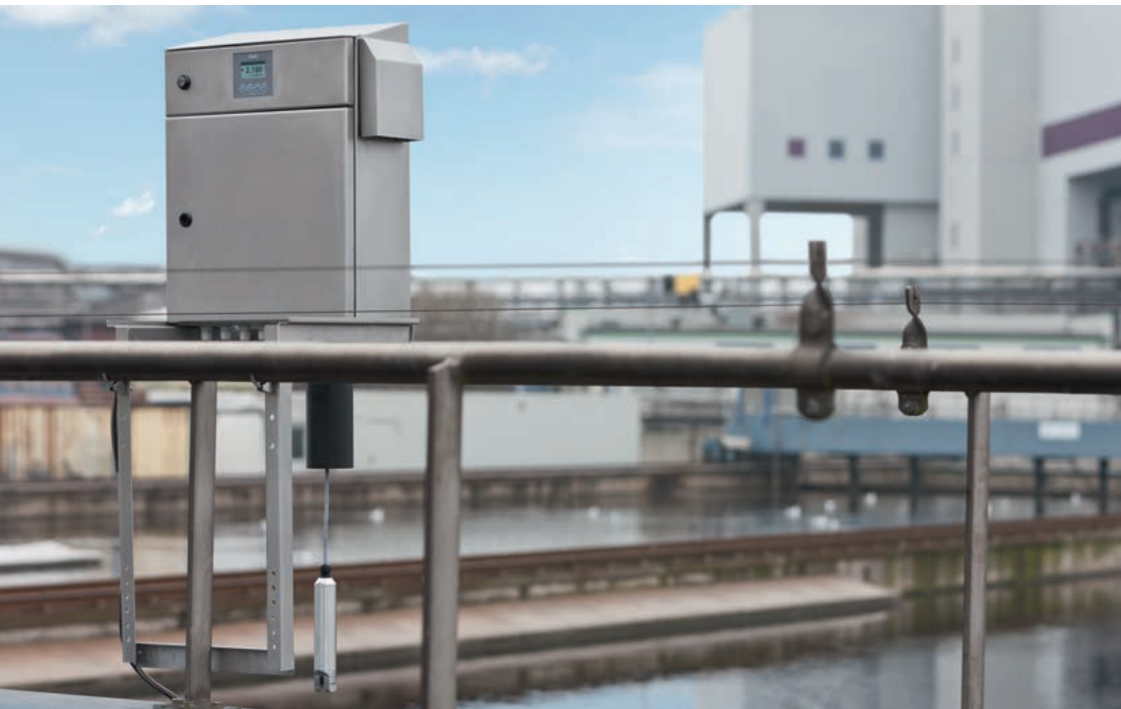
Sludge blanket measurement in secondary clarifier of wastewater treatment plant, Krefeld, Germany
