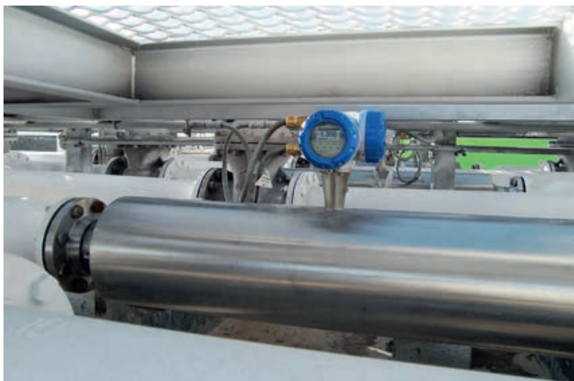
OPTIMASS 2000 – Minimal installation footprint
